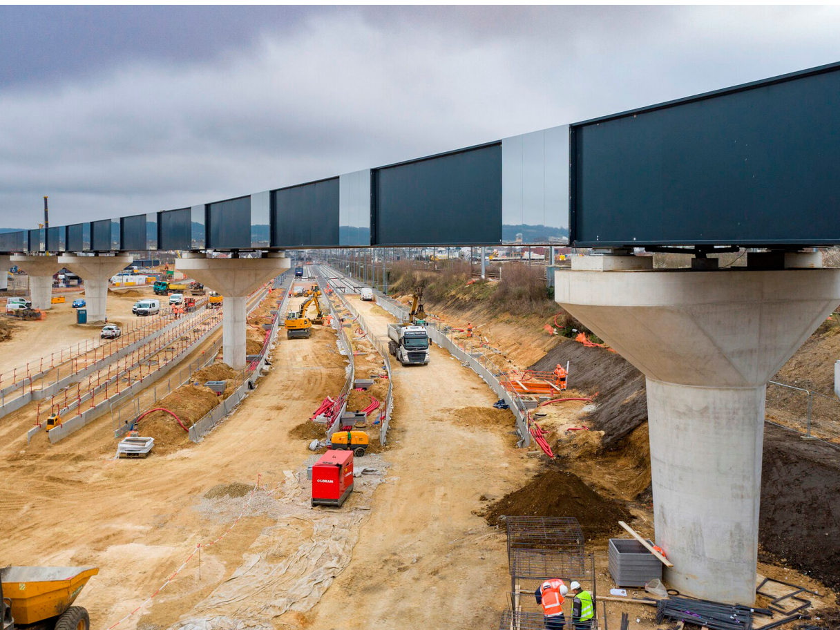
View of the bridge from the abutment
