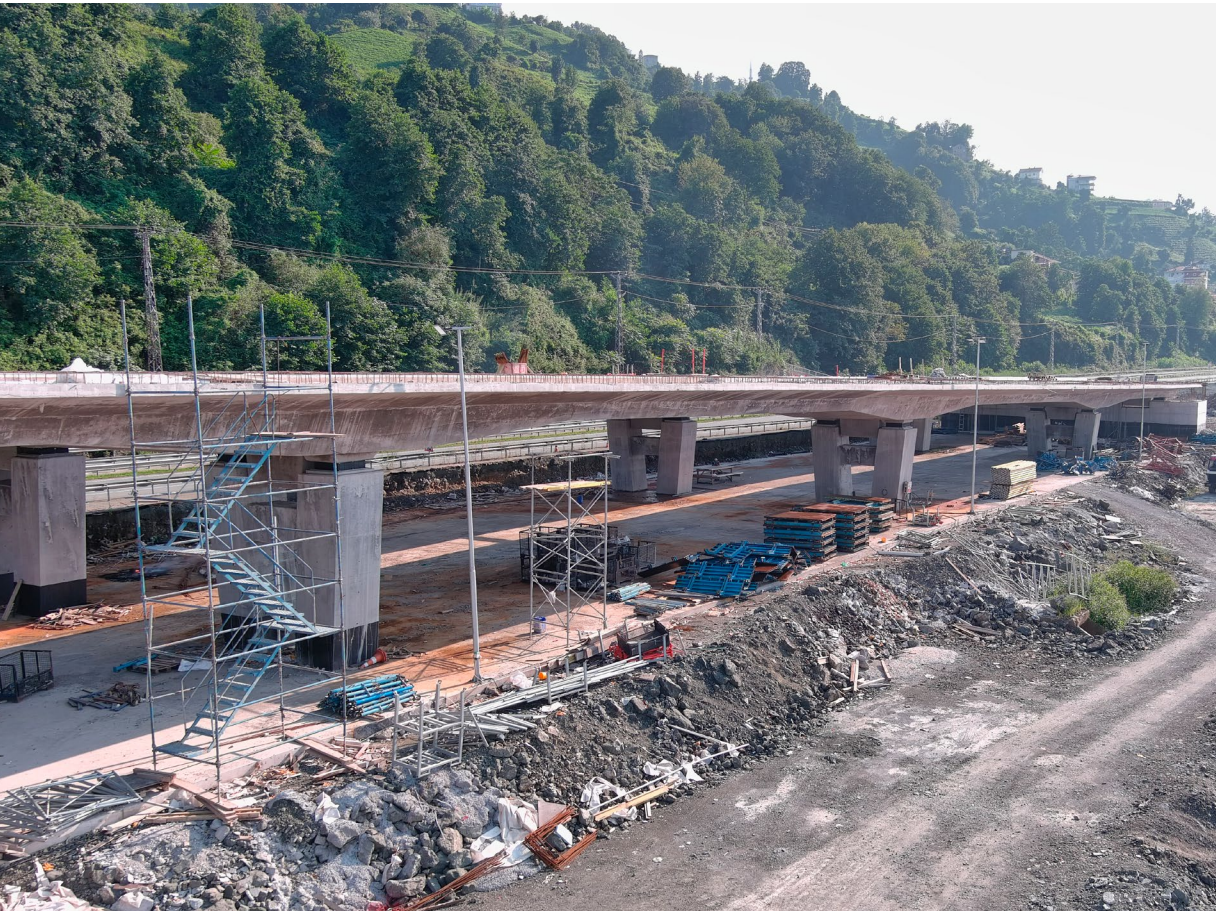
Rize-Artvin Airport Bridge, Turkey
