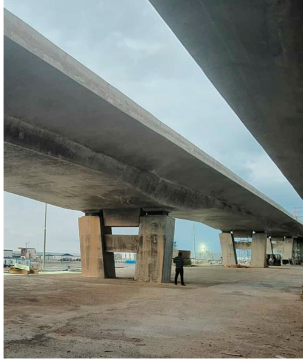
Rize–Artvin Airport Bridge
